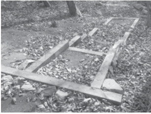
New timber framed steps at the entrance to the Neck River Uplands North trail, the Eagle Scout project of Stephen Hansen.
